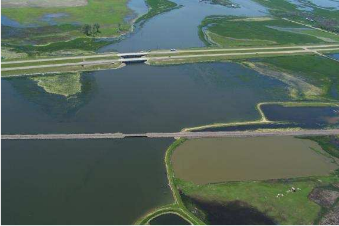
Bridges of the BNSF and U.S. Highway 2.
